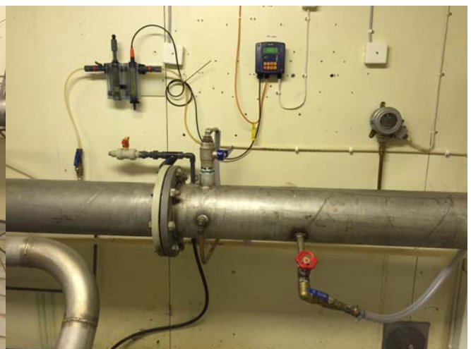
Analyte injection point
