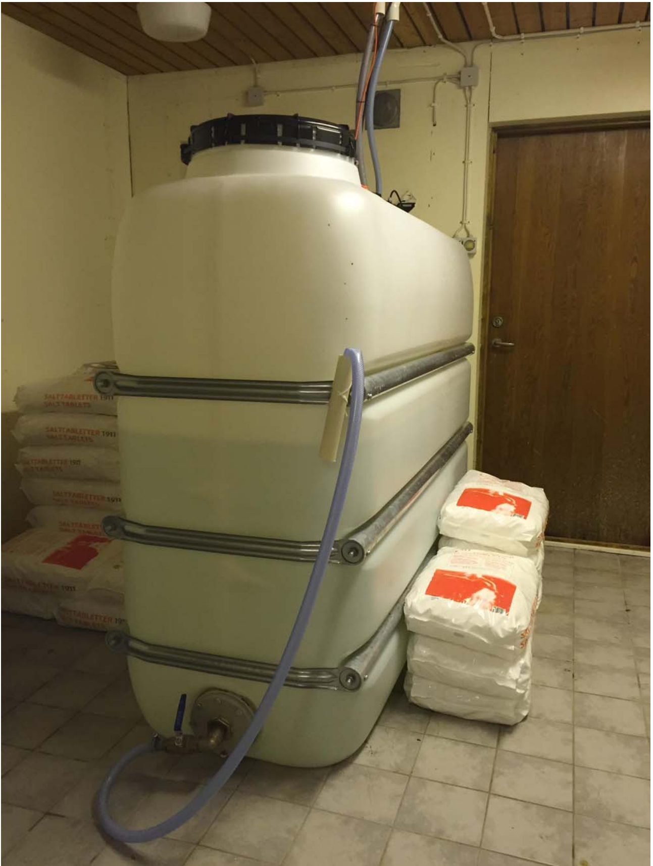
Anolyte storage tank
