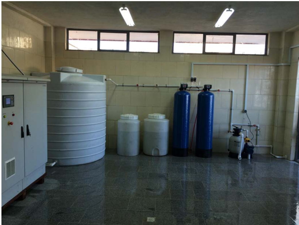
ELA-10 000ANW with brine and anolyte storage tanks, water softeners and dosing pump. Dosing 2 ppm at the injection point.
